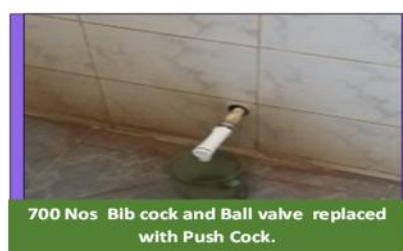
Figure 12. Replacement of BIB cock with push cock.
