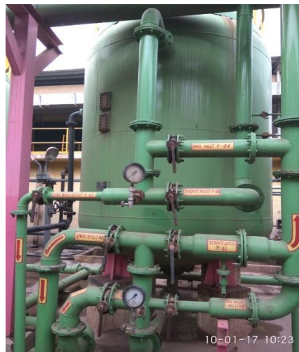
Figure 14. COC optimization and backwash implementation.
