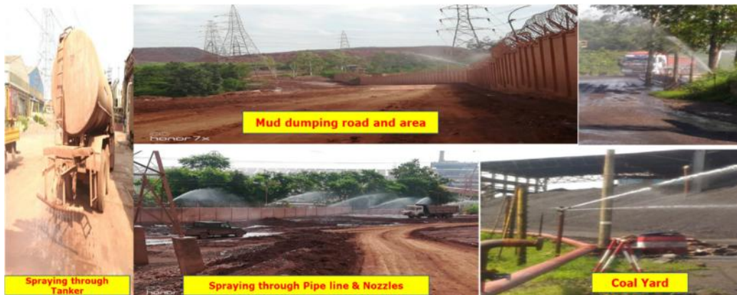
Figure 16. ETP treated water for dust suppression.
