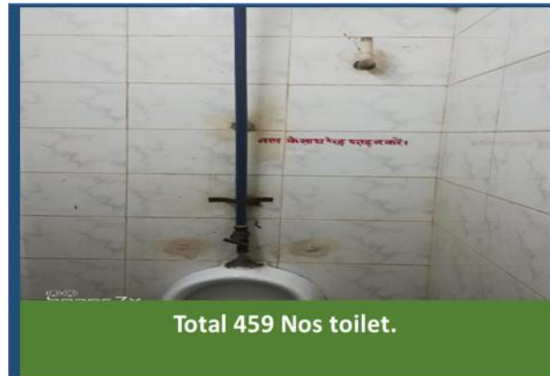
Figure 13. Replacement of drinking water with ETP treated water.
